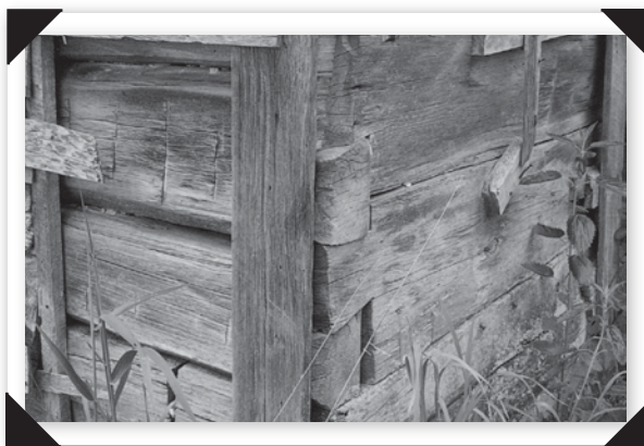
Arley Engle took this close-up photo of hand hewn beams and dove-tail construction at the old Fisher School building
