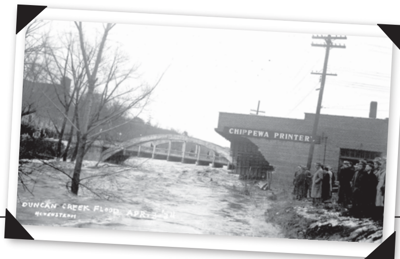
This bridge was the only Duncan Creek bridge that survived the destructive flood of 1934.
